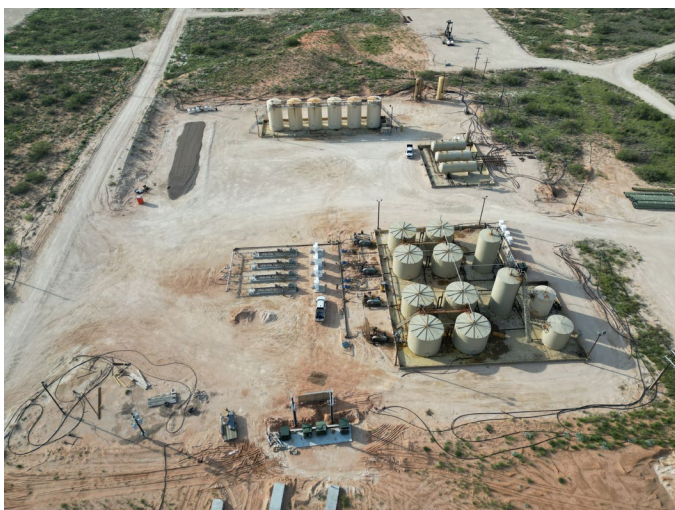
Figure 1. Natural gas processing site.
